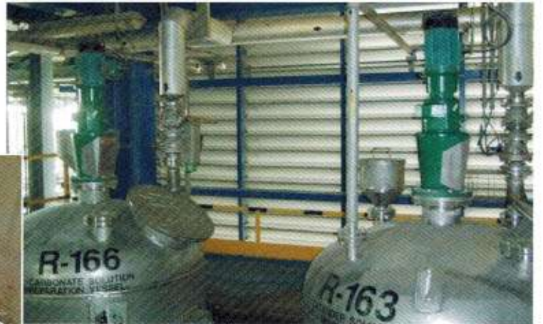
Chemical plant. Malaysia
