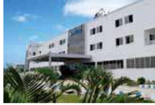
Rudrapur Plant (Green Building)
